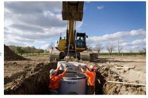
Extended 400E between 200S and Cobblestone Lane, while installing underground water, sewer and storm water infrastructure towards Perrett Park and looping with infrastructure in StoneGate Meadows.
