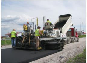
Based and crowned roadway, installed curbing and gutters and paved these two stretches of roadway to improve accessibility to adjacent property owners. This is also part of Council's long term plan to pave every street within the community.
