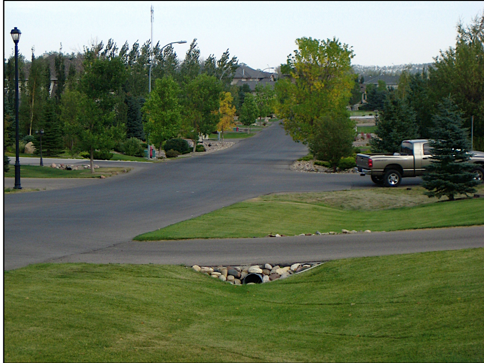
Similar road design in Sandstone Ridge south of Lethbridge.
