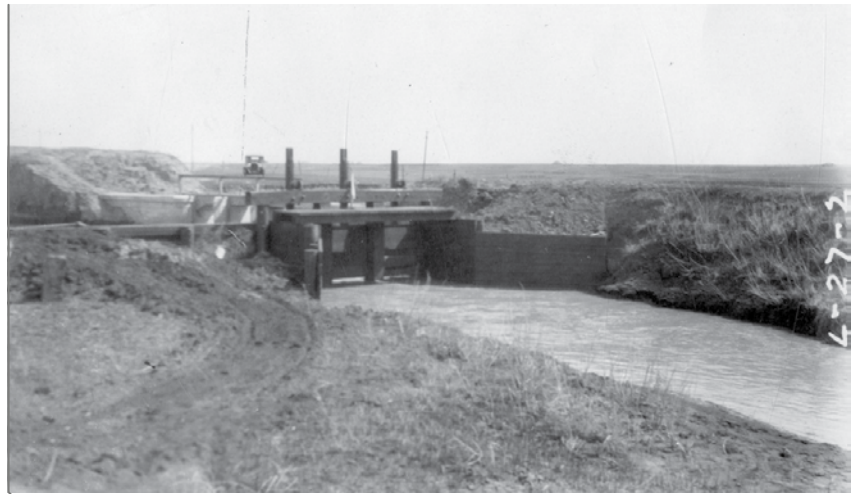
Headgates of the Raymond Lateral, reconstructed in 1927 Canadian Pacific Railway. Department of Natural Resources. Annual Report of Operation and Maintenance - Lethbridge Section. 1927 Galt Archives 1987008010
