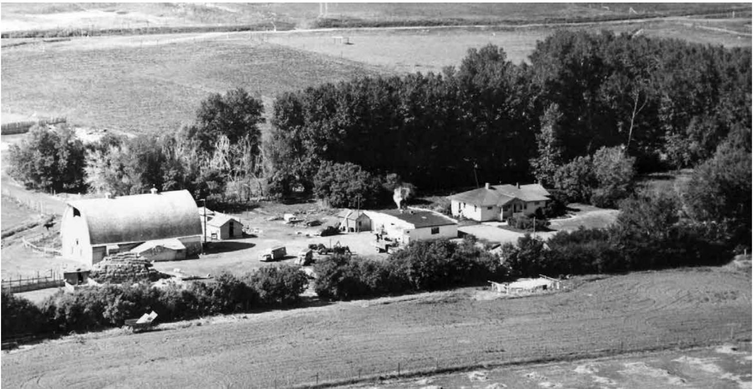
Aerial view of Hancock Dairy landscape, as it appeared in 1952.
