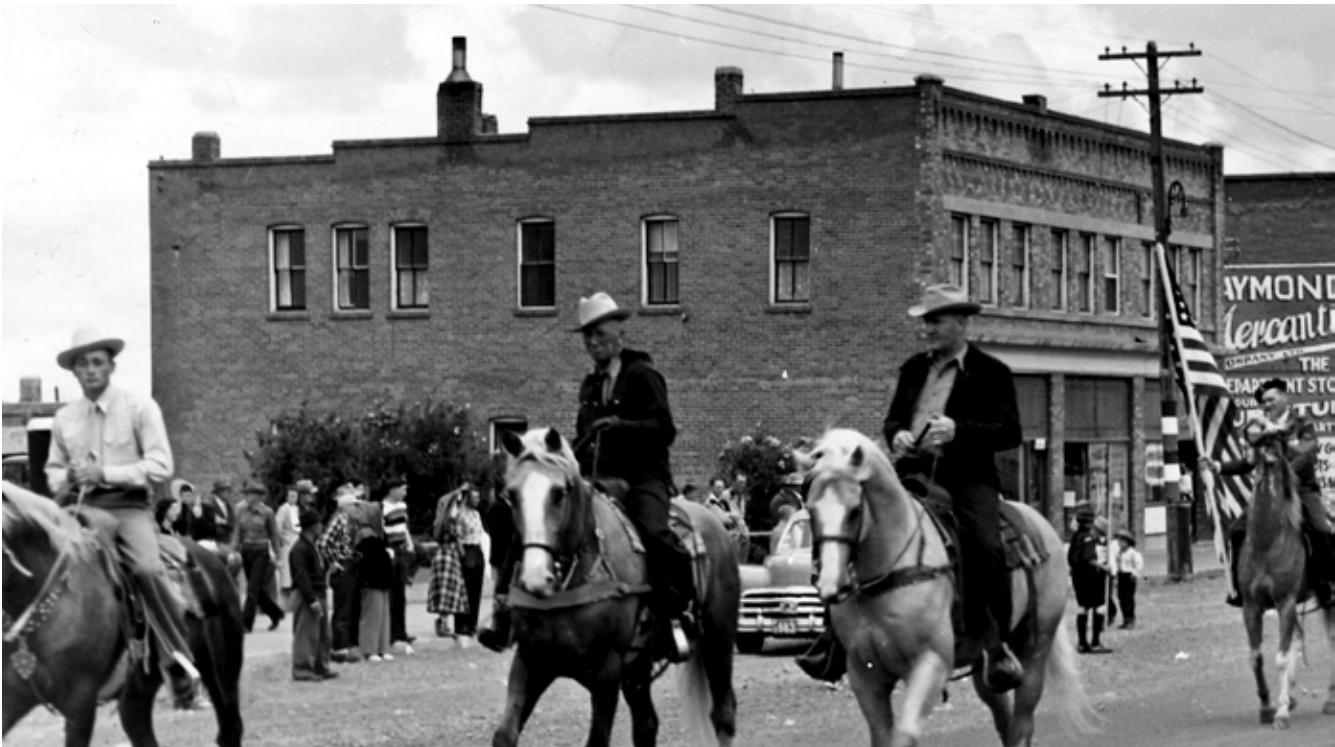
The Post Office Building as it appeared in 1950. Galt Archives P19760209056
