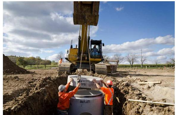
Extended 400E between 200S and Cobblestone Lane, while installing underground water, sewer and storm water infrastructure towards Perrett Park and looping with infrastructure in StoneGate Meadows.
